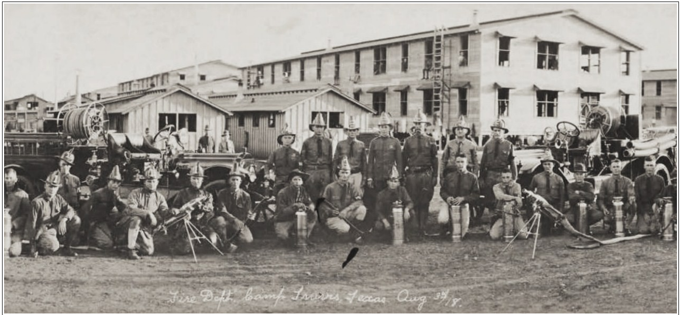
Camp Travis Fire Department – August 1918
