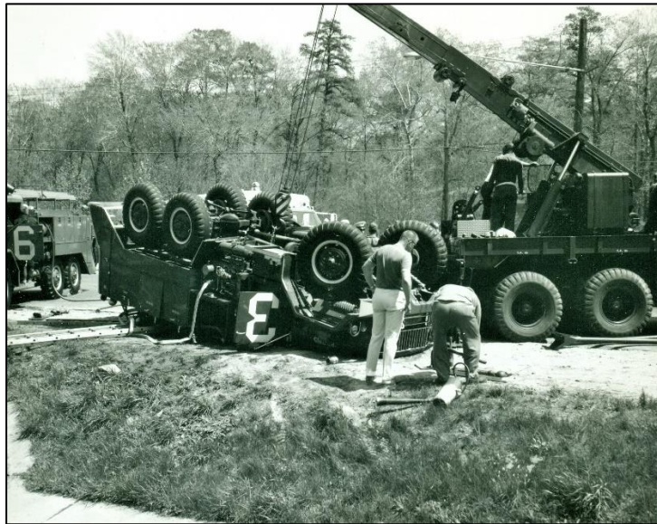
Army crane prepares to upright the truck.
